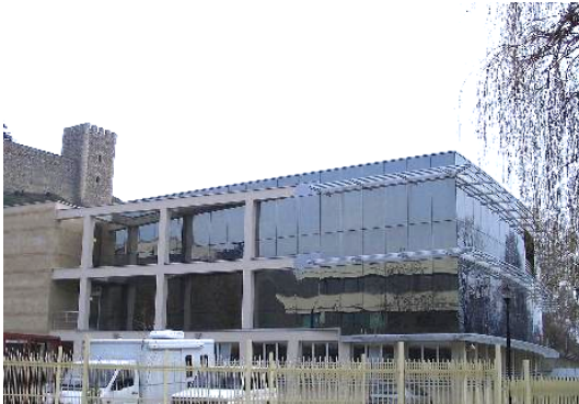
MCA Headquarters second (new) building, hosting the IT and Statistics Department
